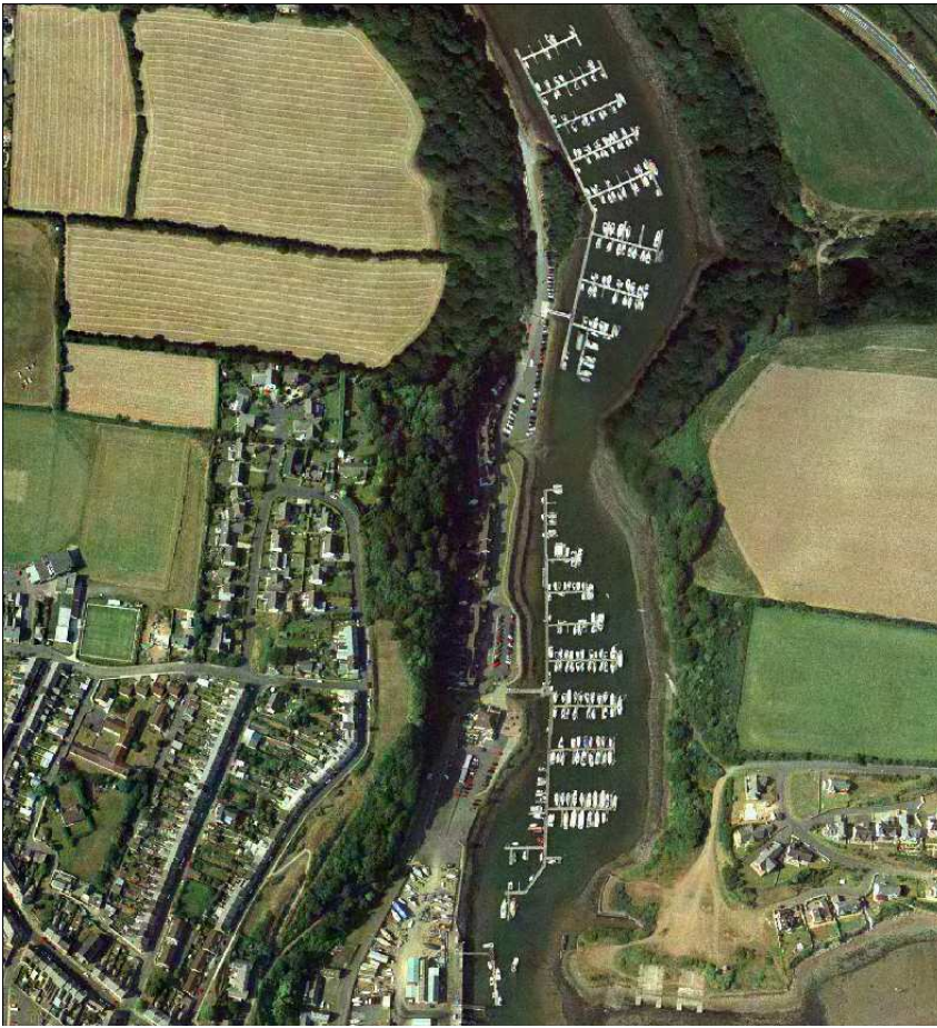
Figure 3 Neyland marina showing the pontoons and finger pontoons
