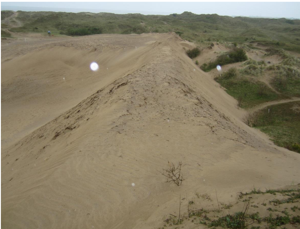
Photo 10. Placement of sand and turfs to enlarge the northern ridge
