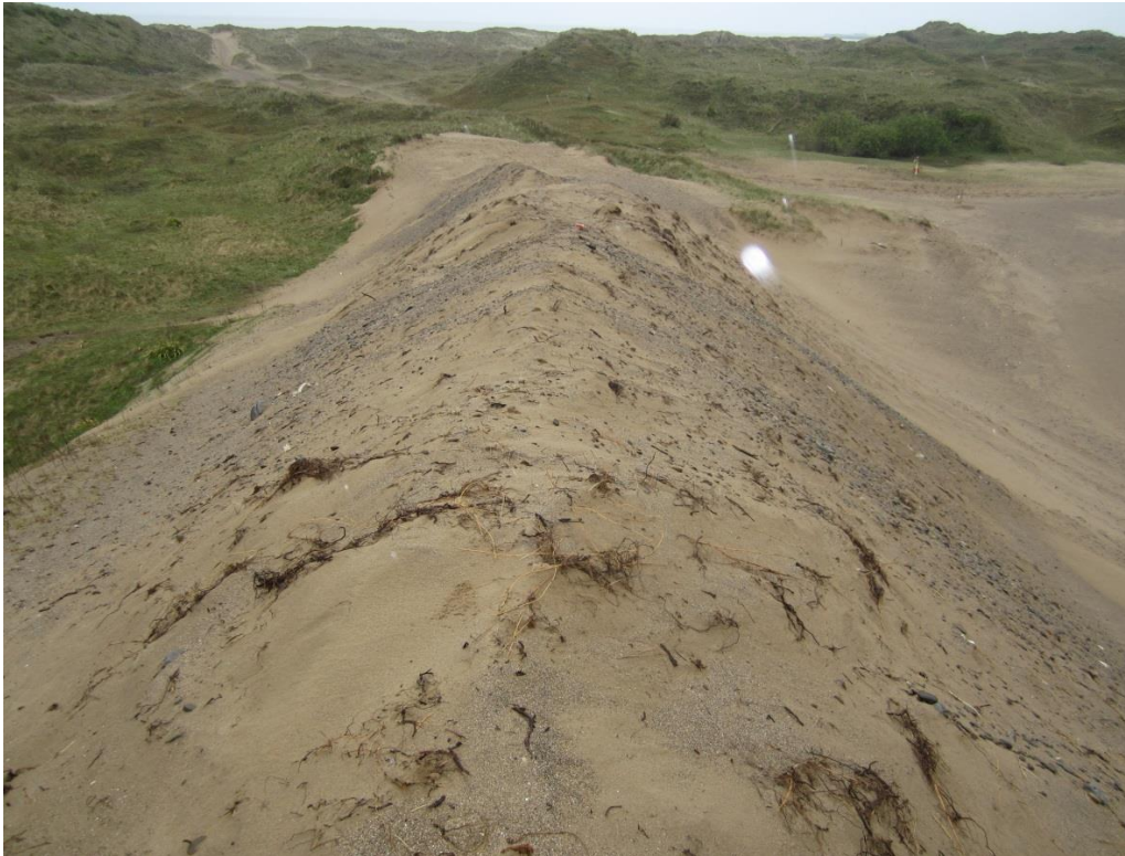
Photo 9. Placement of sand and turfs to enlarge the southern ridge
