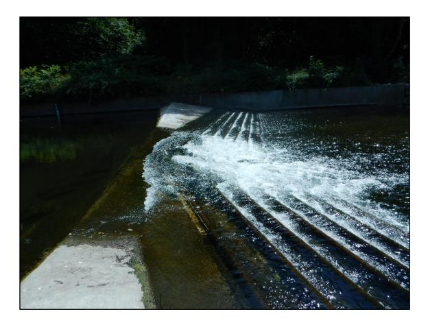
Low Cost Baffle (LCB) solution at Resolven gauging weir – River Neath 2017
