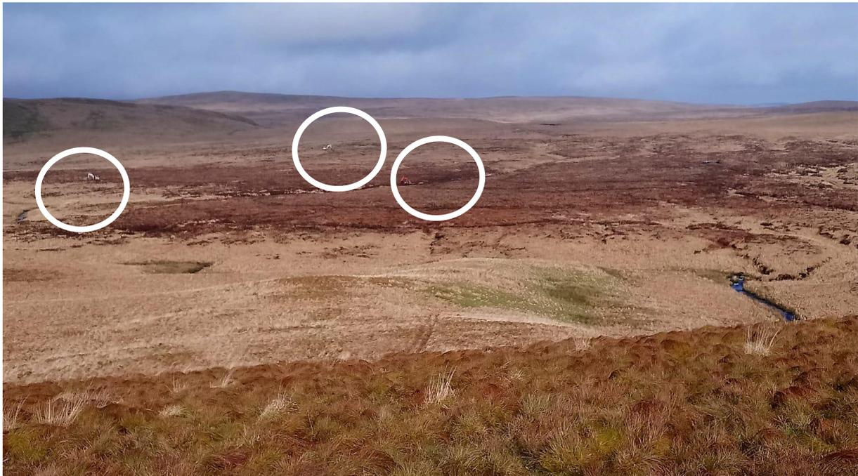
**Figure 6.** Large-scale gully blocking and reprofiling and low elevation contour bunding underway at Waun Figyn at Claerwen NNR which forms part of the Elan Valley Trust Estate. Three excavators (encircled) emphasise the significant scale of this project. Photo: Andy Polkey.
